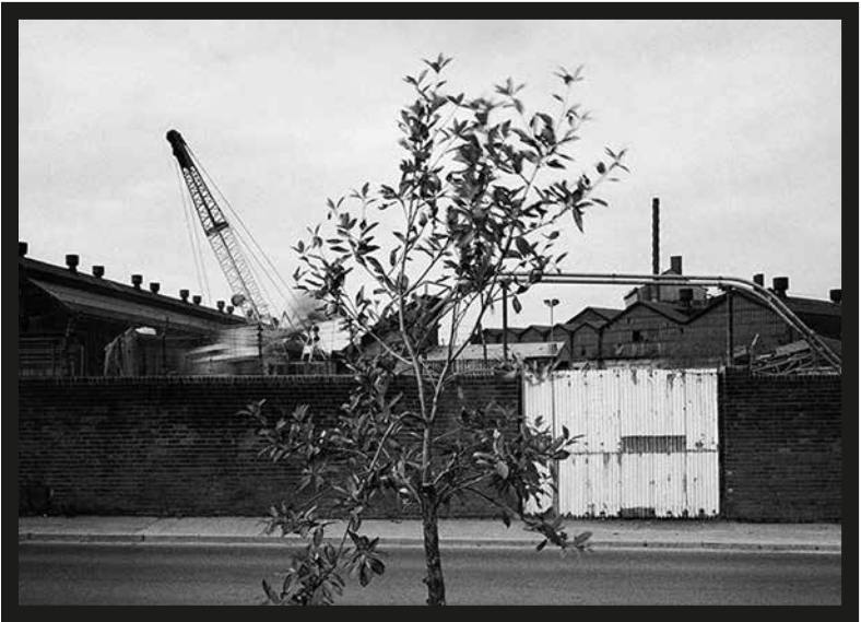
Factory Demolition, Carbrook Street (1989) [John Darwell]
